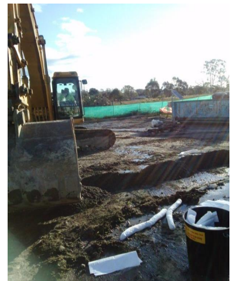
Making a dam with an excavator
